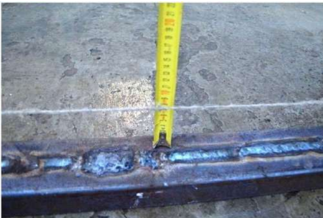
Fig. 3.8. Measurement of deflection in mid-span
