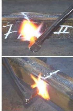
Fig. 3.12. Heating of wedges with gas burner
