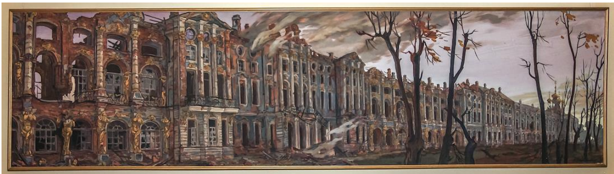
Figure 2. Panoramic picture. It shows the palace in a terrible state in 1944. The canvas reminds us how much damage the 1941-1945 war caused to the Catherine Palace of Tsarskoye Selo
