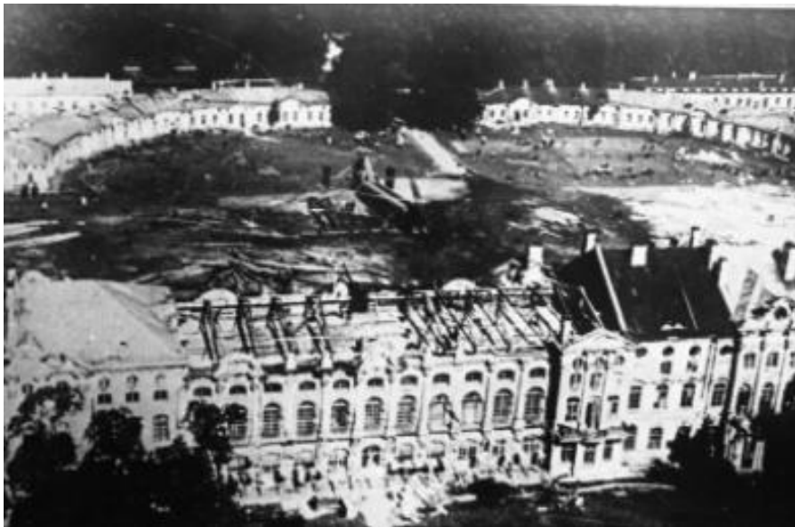
Figure 12. Catherine Palace. The Great Hall area during the trusses' replacement on June 17, 1959. View from the YAK-24 helicopter
