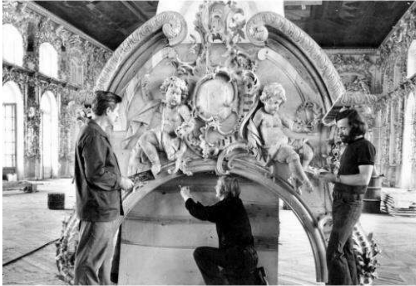
Figure 23. The doorway of the southern wall of the Great Hall after the restoration of the carving before installation on a historical site.
