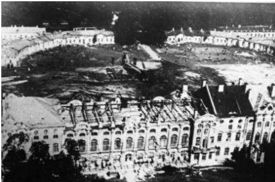
Figure 12. Catherine Palace. The Great Hall area during the trusses' replacement on June 17, 1959. View from the YAK-24 helicopter
