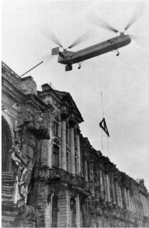
Figure 13. Installation of new trusses over the Great Hall on June 17, 1959. Helicopter commander I.S. Grigoriev
