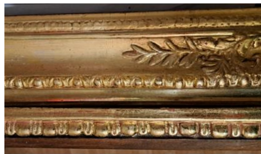
Figure 19. Tinting of matte gilding scuff areas on matte gilding loss areas and glossy gilding restoration on the door frame egg-end-darts
