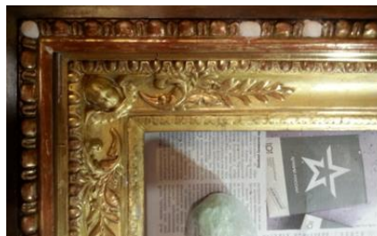
Figure 11. Reconstruction of local losses of mastic decor in the left part of the door frame. Installation of recreated mastic decor fragments at the place of local losses of the author's decor
