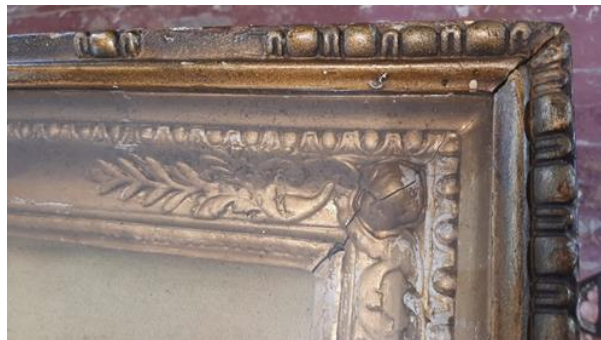
Figure 5. The loss of the mastic stucco decoration of the egg-and-darts on the outer frame-door and the divergence of the "moustache" joints of both frames in the corners
