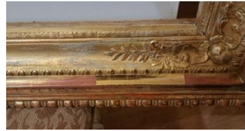
Figure 15. Trial gilding on the polymer on the outer listel of the inner icon frame in the severe abrasion area (right). The icon frame fragment with polished gold on the outer frame pull
